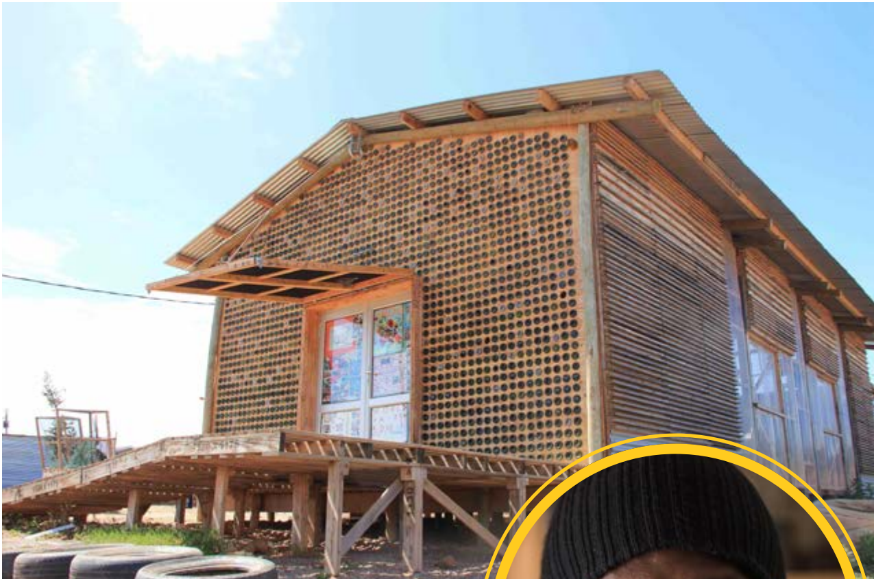
The Silindokuhle Preschool, designed by Kevin Kimwelle, is built from bottles and recycled wooden pallets. Kimwelle's work is featured on the Common Good First online website.
